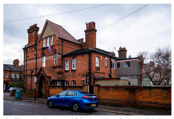
**Figure 37** Rear extensions of the terrace on north Gladstone Avenue, looking west from Darwin Road. Red circled area shows the extension on the first two properties. Also note the alterations to the original closet wing windows (SLHA@Dec'21).
